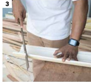
3 Cut the moulding to the required length and angle by using manual tools
