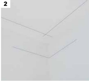
2 Mark the dimensions and locations on the wall surface
