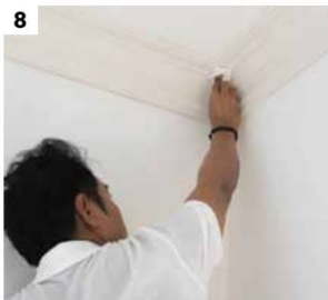
8 Immediately after the moulding is installed on the wall surface, wipe off all the putty A,B glue extruded outside of the moulding while they are wet
