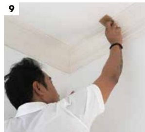
9 After the putty dry up completely smoothen the connecting areas to level with sandpaper. Then apply paint on the surface
