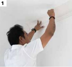
1 Mark the moulding location by drawing dimensions lines on wall and ceiling
