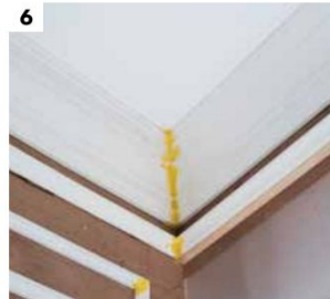
6 There should be 1-2mm juncture between moulding, then fill with white cementing compound or liquid nail during installation (modified the surface of moulding with bounded knife)
