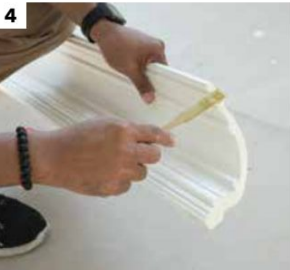
4 Apply white cementing compound or liquid nail on the contact surface between the moulding and wall surface and between moulding
